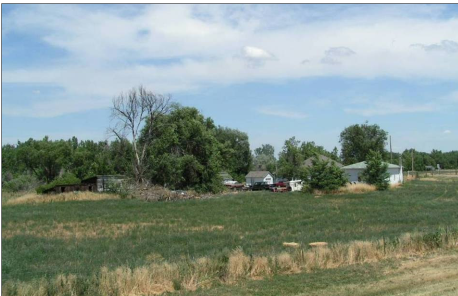
Swinburg Farm, 5BL.10405, an increasingly rare example of intact farm buildings on agricultural acreage, was bisected diagonally by construction of the U.S. 287 bypass.
