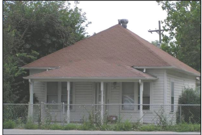
Adams House, 5BL.10397, is one of Lafayette's most intact examples of the Hipped-Roof Box that proliferated during the coal mining decades.
