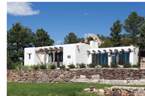
The Heller main house was restored in 2010
