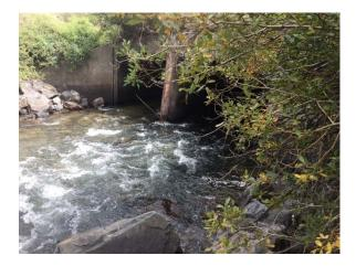
**Photo 6.** Looking southeast at perennial stream S-1F (i.e., Clear Creek). Note the large concrete box culvert that conveys water south and under I-70.
