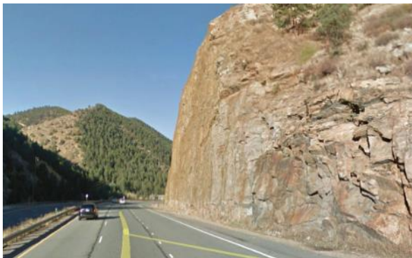
Photo 5. Rock Stabilization at MP 237.1 Source: Google Earth 2015.
