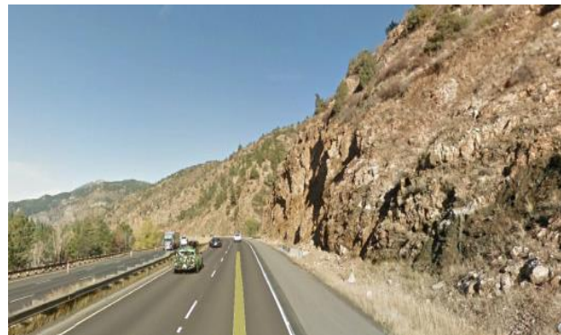
Photo 6. Rock Cut and Stabilization at MP 236.4 Source: Google Earth 2015.
