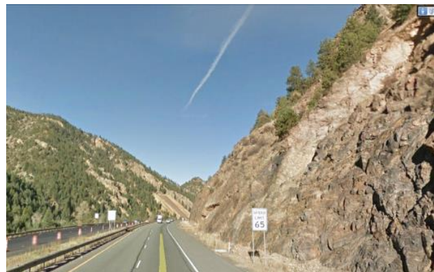
Photo 3. Rock Stabilization at MP 238.4 Source: Google Earth 2015.
