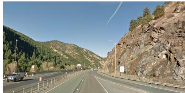
Photo 1. Exit 239 On-Ramp to Fall River Road Source: Google Earth 2015.
