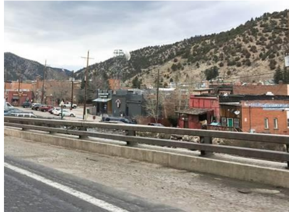
Photo 10. Example of Type 10 Barrier Rail
