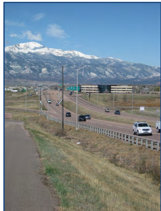
US 24 at Powers Boulevard (SH 21)
