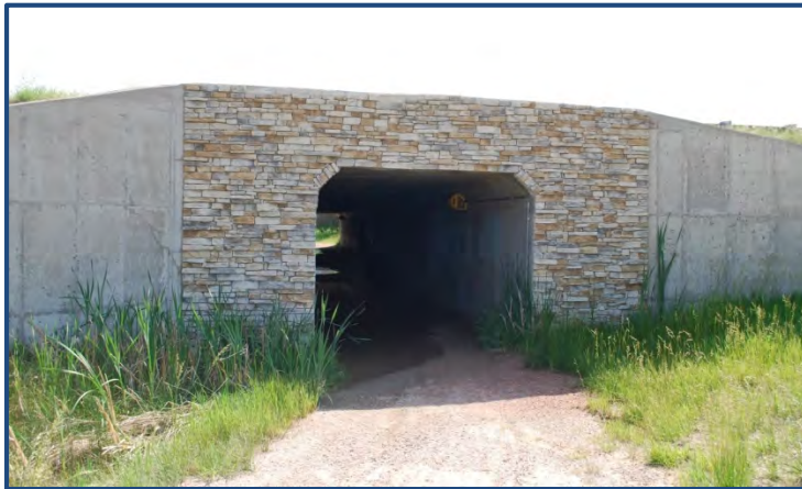
Rock Island Trail underpass at Woodmen Road
