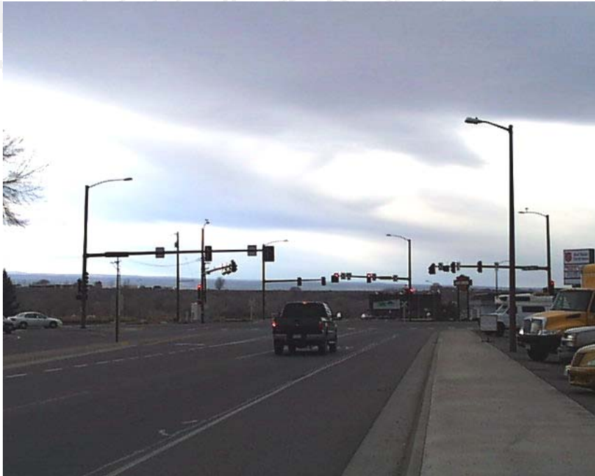
Intersection of San Juan Avenue/Townsend Avenue (U.S. Highway 50) looking west. (Rear-end accidents in the right turn lane shown here (turning right from San Juan Avenue onto Townsend Avenue) are the majority of accidents (68 percent) that have occurred at this intersection since January 1, 2007.) (Photo taken December 14, 2010.)
