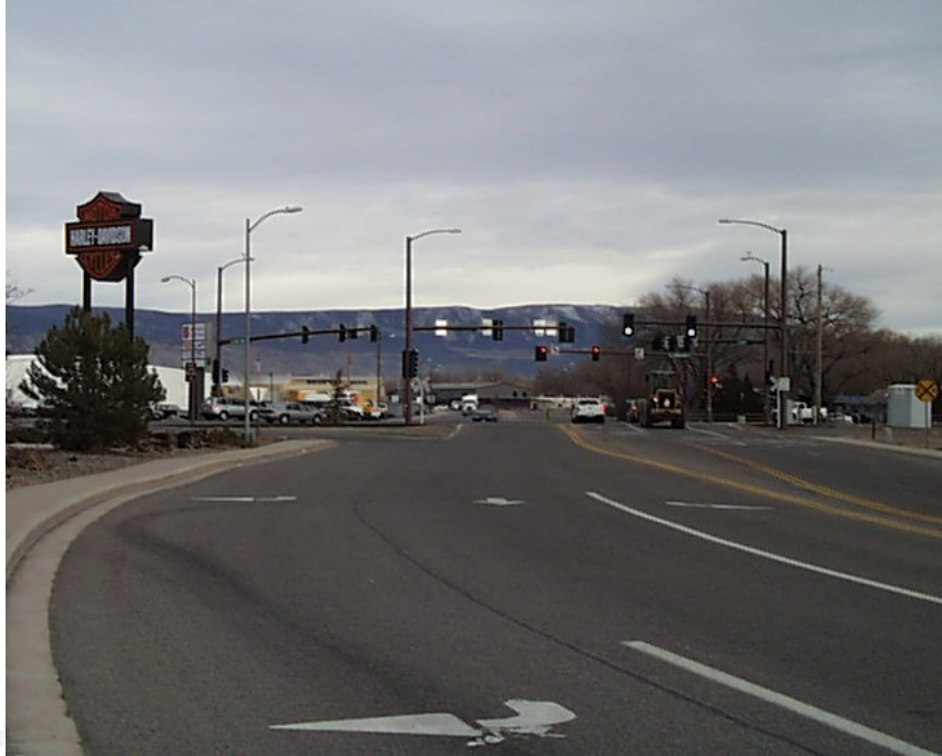
Intersection of San Juan Avenue/Townsend Avenue (U.S. Highway 50) looking east. (Photo taken December 14, 2010.)
