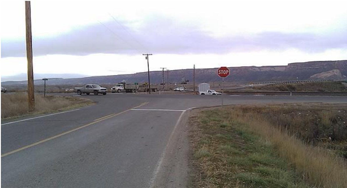
Intersection of 20 Road and Highway 6, looking south along 20 Rd. Misalignment in intersection can be seen (dump truck is attempting to turn west onto highway from 20 Rd.)
