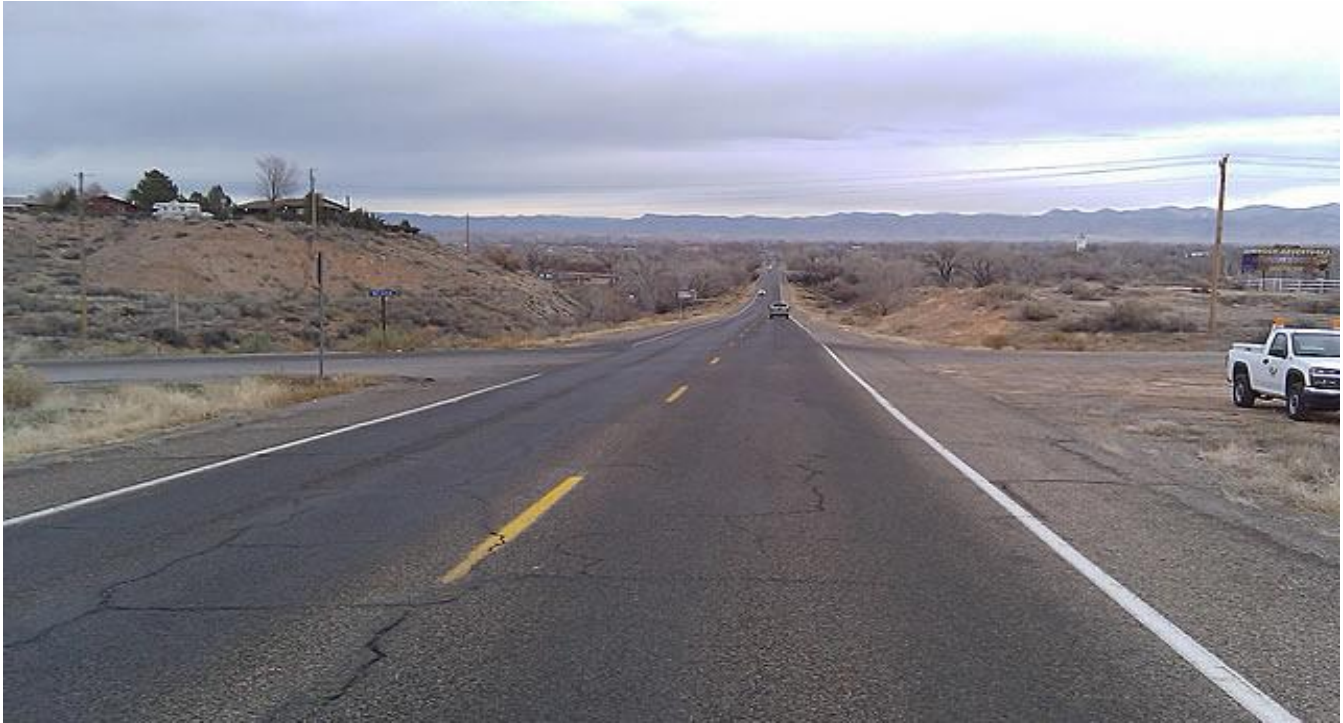
Intersection of Kingsview Road and Highway 340, looking north. Note lack of accel/decel lanes and narrow width of highway in this location.
