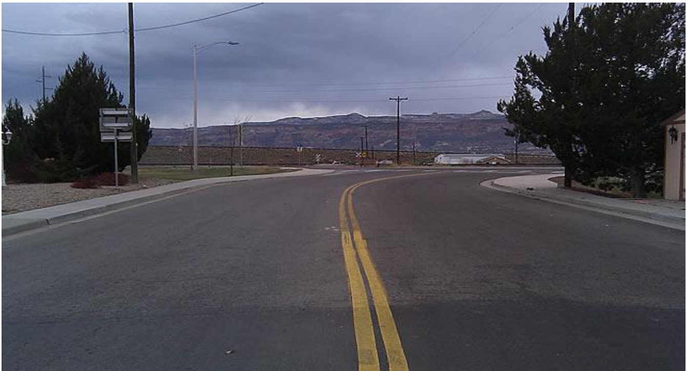
Intersection of 17 Road and Highway 6, looking south. Realignment of 17 Rd. north of highway is apparent in this photo. Note the railroad crossing signs south of highway. These signs straddle the alignment of 17 Road south of Highway 6.
