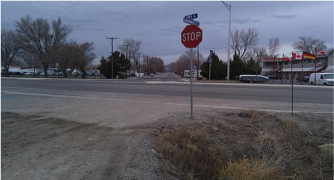
Intersection of 17 Road (Greenway Dr./Coulson St.) and Highway 6, looking north. 17 Road north of highway has been realigned to intersect Hwy. 6 at a 90° angle. Misalignment of north/south street is apparent in this photo.
