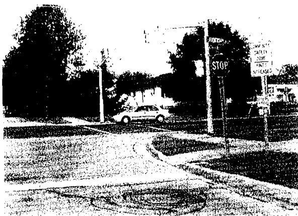
Figure 7-3B. Intersection pedestrian signals in Portland, Oregon, and the Puget Sound area. (Source: top: William C. Kloos; bottom, Randy S. McCourt, Portland, OR, USA.)
