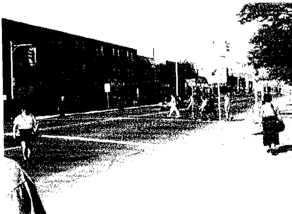
Figure 7-2A. Midblock signal-controlled crossing in Toronto, Ontario, Canada. (Source: Douglas Allingham, Whitby, ON, Canada.)
