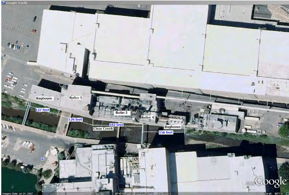
Figure 2: Aerial Zoom of CENC Facility
