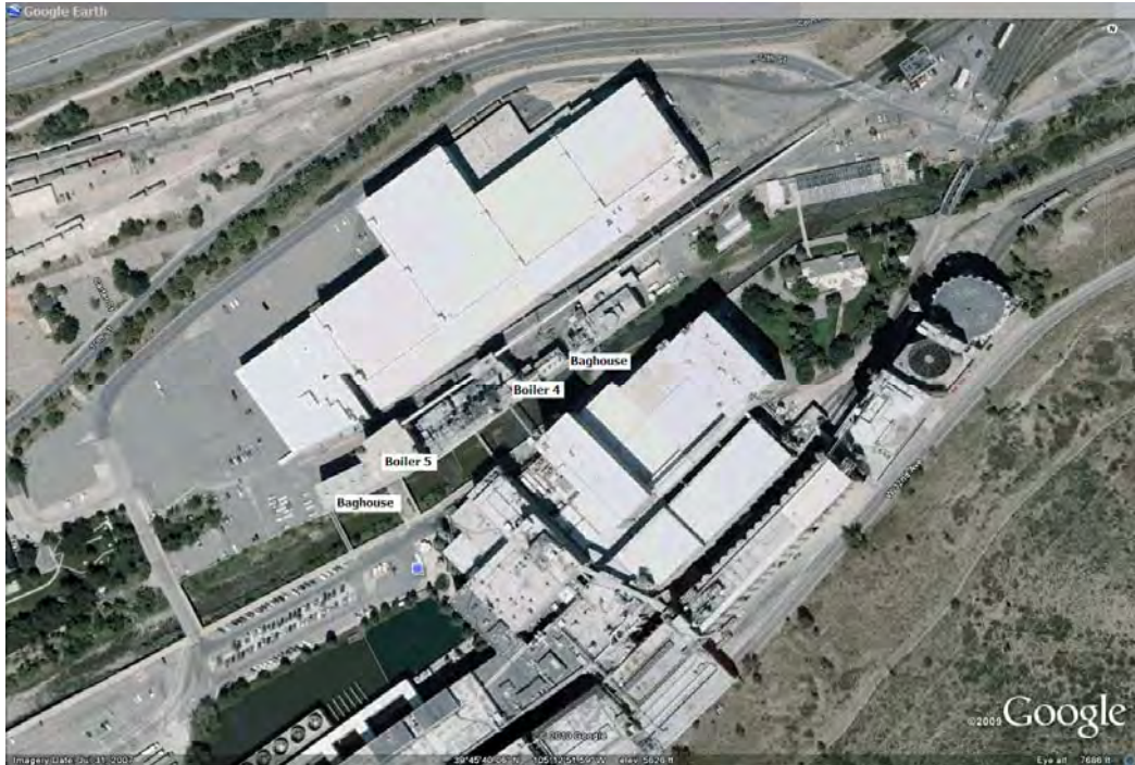
Figure 1: CENC facility Aerial Perspective
