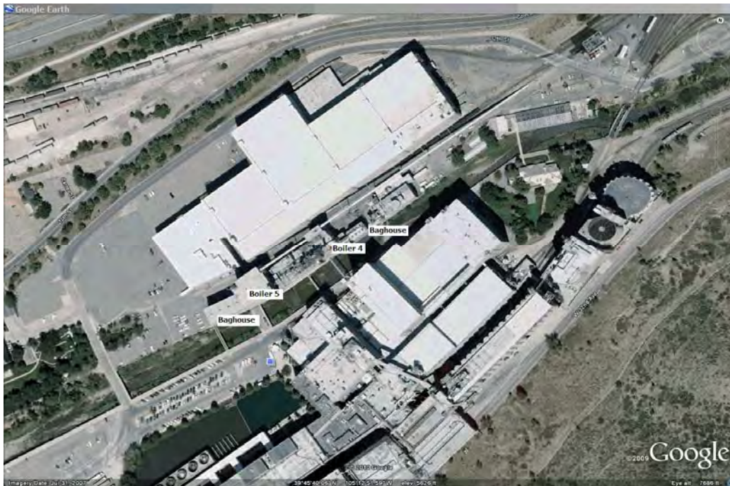
Figure 1: CENC facility Aerial Perspective
