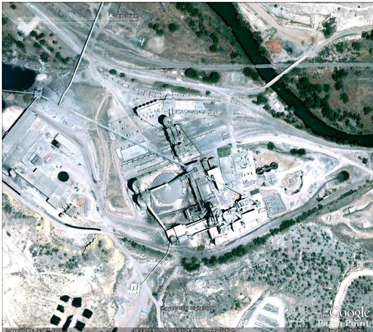
Figure 1: Holcim Portland Plant Aerial Perspective
