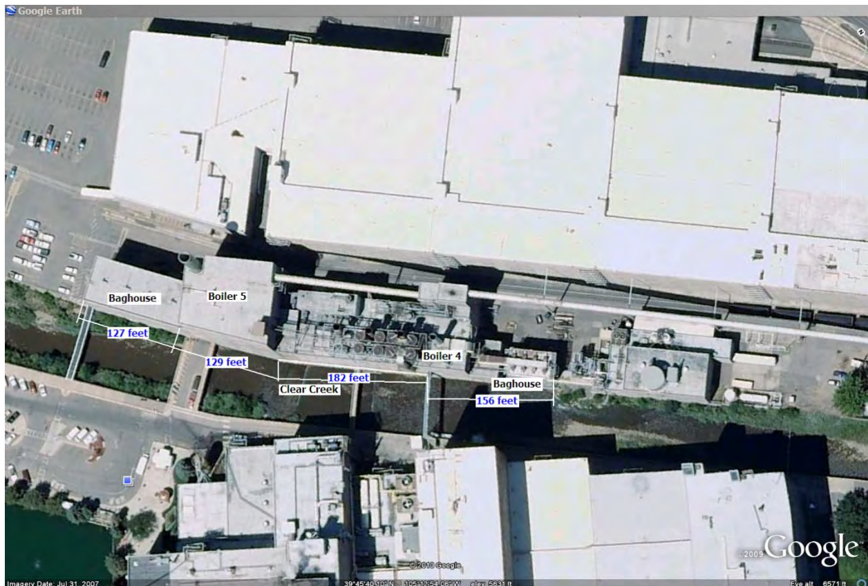
Figure 2: Aerial Zoom of CENC Facility
