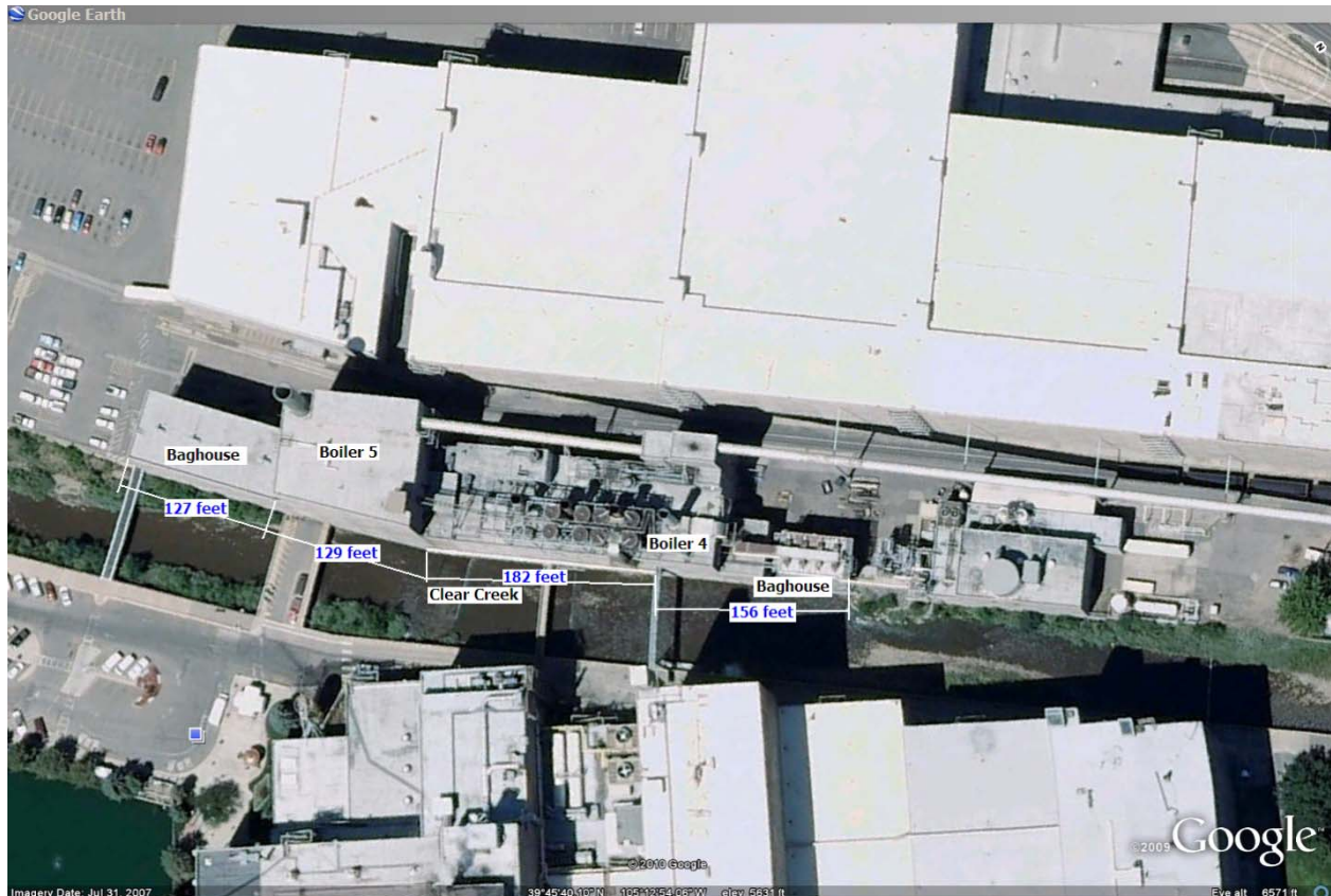
Figure 2: Aerial Zoom of CENC Facility
