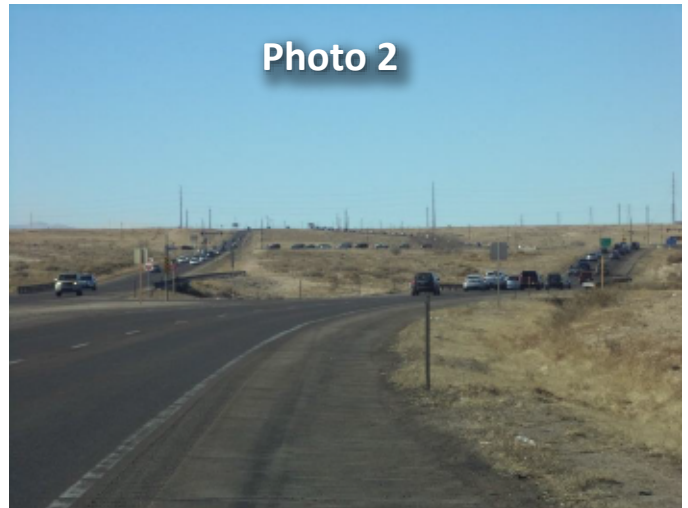
View of US 50 rural corridor to Pueblo Blvd, photo taken 1/26/2014.
