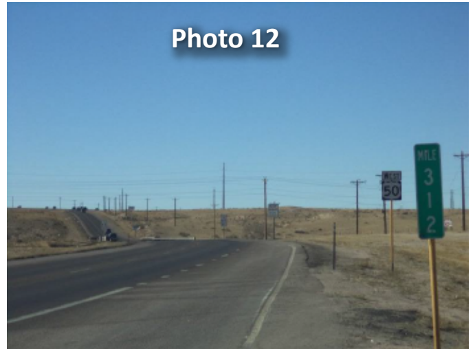
Milepost 312 is just past Pueblo Blvd, photo taken 1/26/2014. View of continuous rural corridor until Purcell Blvd.
