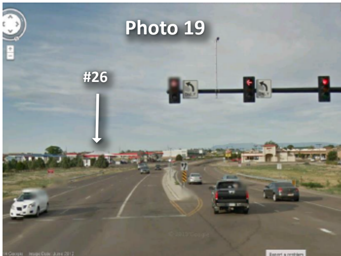
Looking south on Purcell from US 50, Loaf and Jug #85 (GeoSearch Site 26) with retail stores in the background.
