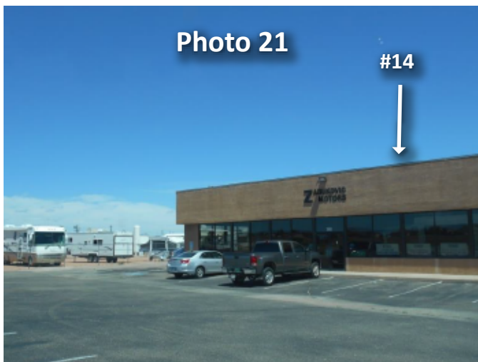
An aboveground storage tank was present at Zabukovic Motors (GeoSearch Site 14). Zabukovic Motors is located south of US 50.
