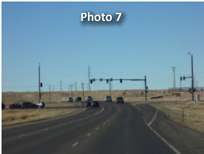
Heading west on US 50 intersecting with Pueblo Blvd.
