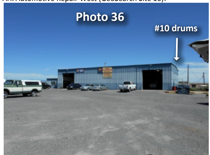
View of Ark Automotive Repair West (GeoSearch Site 10); east of the building is located 55 gallon drums. Located between milepost 208 to McCulloch.
