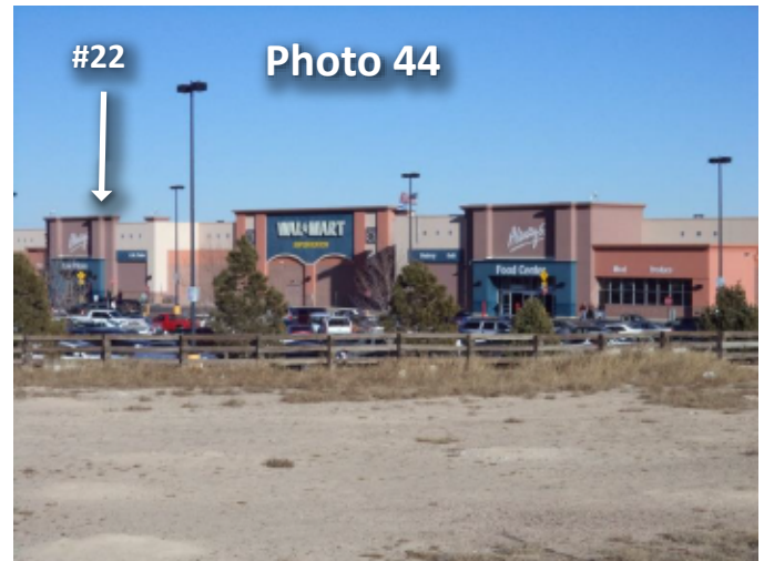
NE corner of McCulloch and US 50 with Wal-Mart Shopping Center (GeoSearch Site 22) in the background.
