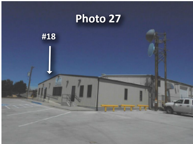
South side view of Tri-State Generation (GeoSearch Site 18) located east of 4 Rivers Equipment and John Deer (GeoSearch Site 20/20B).
