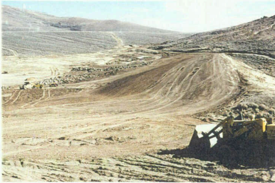
Excavation and Grading Work from the Dams Right Abutment
