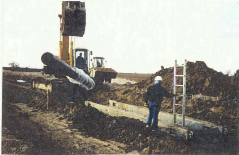
Placement of the 16 inch Diameter - Ductile Iron Pipeline
