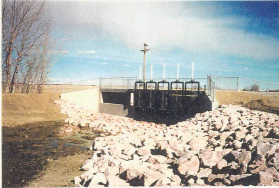
Looking Down/Stream from the Dam at Emergency Spillway/5-Bay Outlet Gate Structure
