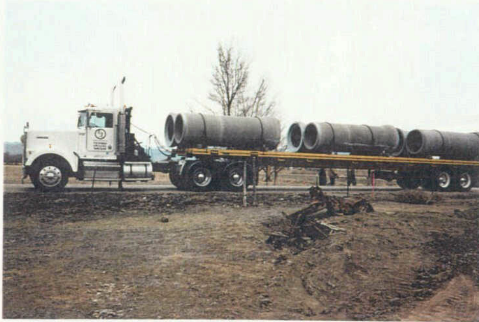
Delivery of the 36 in. Reinforced Concrete Pipe
