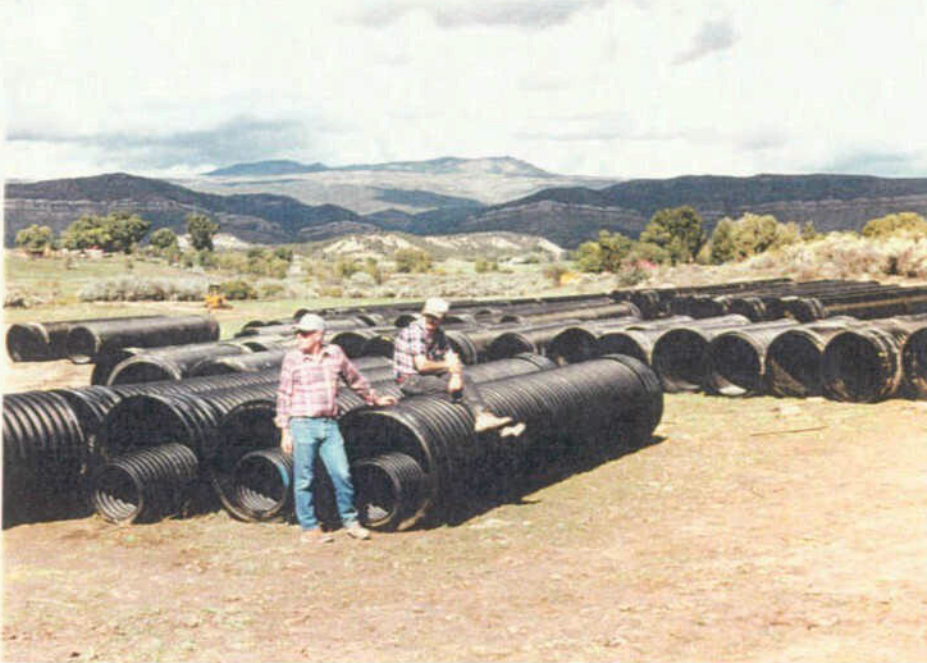
The Owner and Design Engineer Inspecting the Polyethylene Pipe
