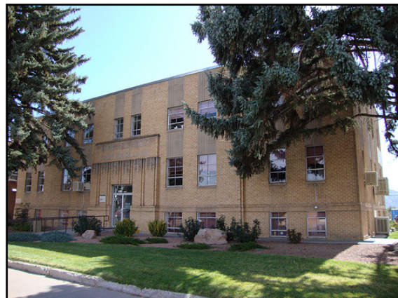
Montezuma County Courthouse, Cortez, CO
