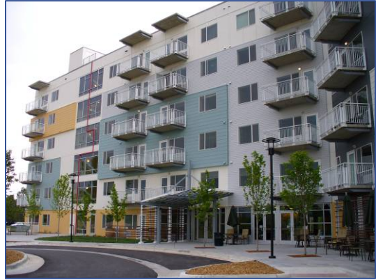
Affordable, multi-family housing funded with program dollars administered by DOLA.
