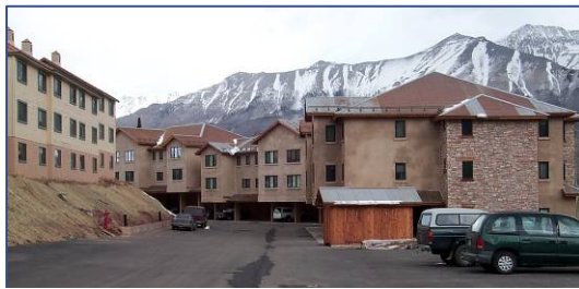
An example of one of many of Colorado's multi-family, affordable housing units made possible through programs administered by DOLA.
