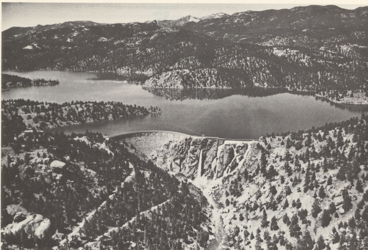
Figure 20. Cheesman Dam and Reservoir, a National Historic Civil Engineering Landmark. (Photo courtesy of the Denver Water Board.)
