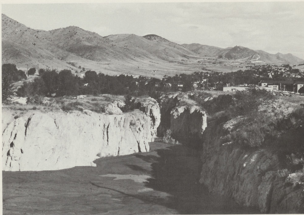
Figure 16. Fly ash slurry disposal as a stabilizing medium for reclamation of abandoned clay pits, Golden, Colorado. The fly ash is delivered by truck, in a wet mixture, over the 15 mi (24 km) distance from the Arapahoe Station of the Public Service Company of Colorado, in Denver. Approximately 3.5 \times 10^3 yd 3 ( 2.7 \times 10^3 m 3 ) are produced and delivered each week in a fleet of ten trucks. Mining of the vertically-bedded Laramie Formation clay strata has been going on since about 1876 by members of the Parfet family, who have been managing the fly ash disposal since 1979. Eventual reclamation of the clay pits is planned, with structural foundations designed to span the slurry fills, bearing on the Laramie interbeds (Photograph by Allen W. Hatheway, September 1980).
