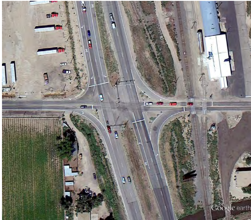
Figure 183 Aerial Photo: US 85L / SH 392A (CR 68) (MP 272.48)
