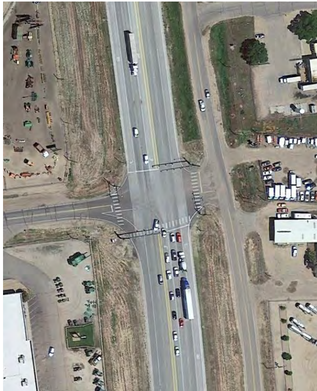
Figure 175 Aerial Photo: US 85L / 5 th Street (MP 268.49)
