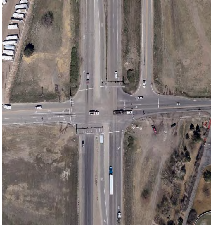
Figure 171 Aerial Photo: US 85L / SH 263A (8 th Street) (MP 268.22)
