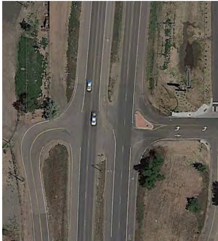
Figure 87 Aerial Photo: US 85C / Denver Street (MP 235.60)
