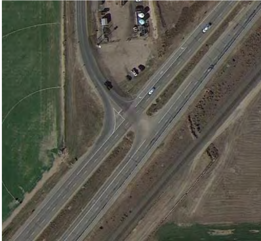
Figure 127 Aerial Photo: US 85C / SH 60 (CR 27) (MP 253.81)
