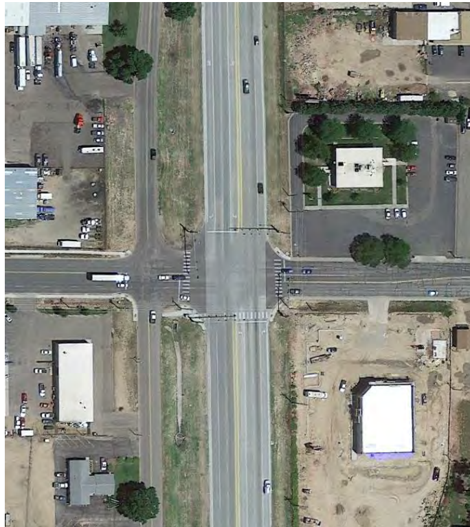
Figure 155 Aerial Photo: US 85L / 22 nd Street (MP 266.65)
