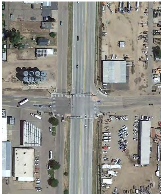
Figure 163 Aerial Photo: US 85L / 16 th Street (MP 267.44)
