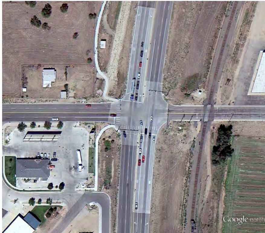
Figure 143 Aerial Photo: US 85C / 42 nd Street (MP 264.11)
