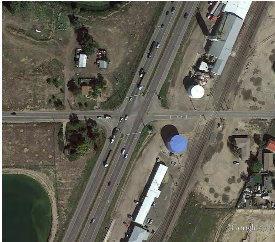
Figure 69 Aerial Photo: US 85C / 124 th Avenue (SH 22A) (MP 230.29 & MP 1.84)
