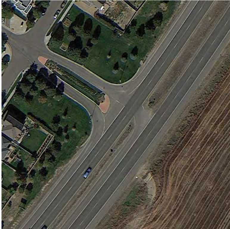
Figure 59 Aerial Photo: US 85C / Long Peak Drive (MP 227.91)
