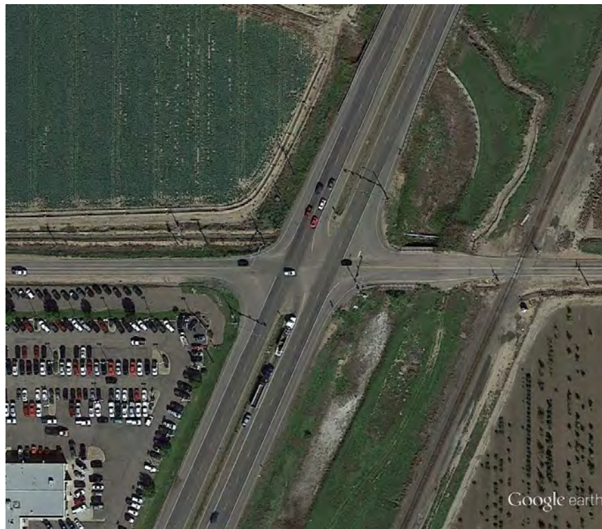
Figure 75 Aerial Photo: US 85C / 136th Avenue (MP 231.93)
