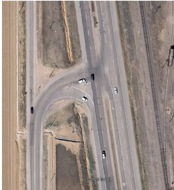
Figure 181 Aerial Photo: US 85L / 11 th Street (MP 271.19)
