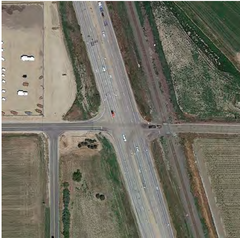
Figure 189 Aerial Photo: US 85L / CR 76 (MP 276.62)
