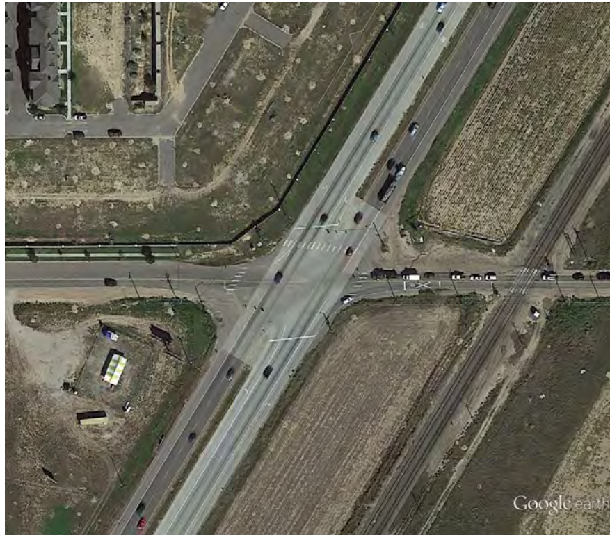
Figure 61 Aerial Photo: US 85C / 112 th Avenue (MP 228.57)
