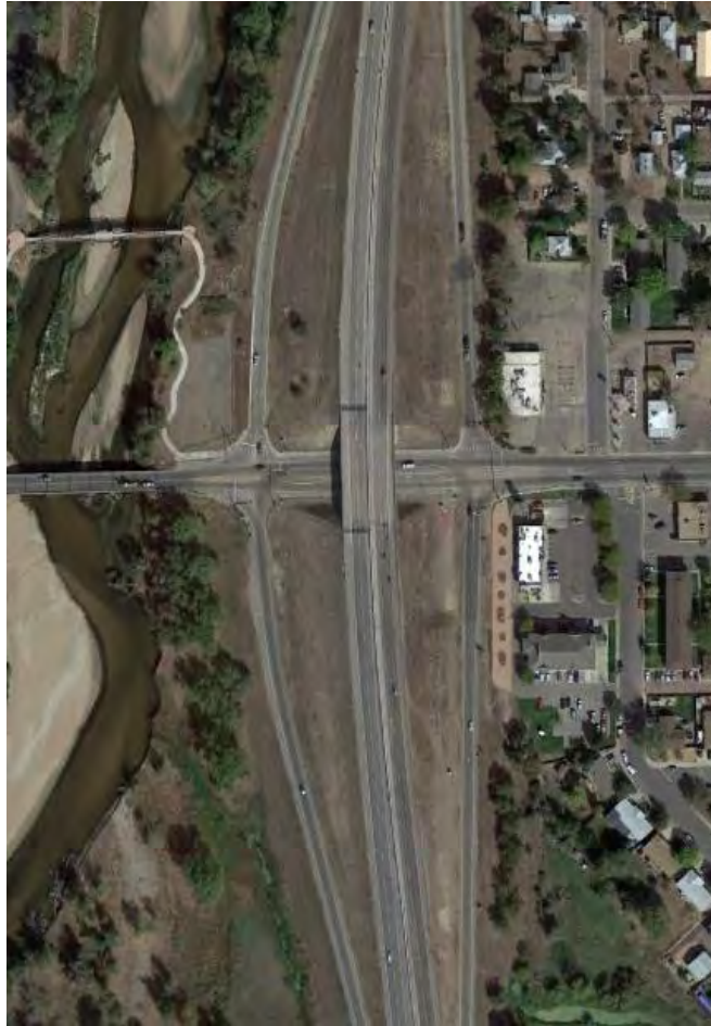
Figure 101 Aerial Photo: US 85C / SH 52A (MP 235.10 & MP 19.96)
