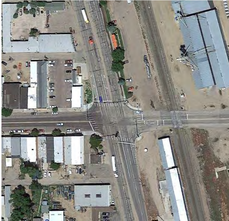
Figure 191 Aerial Photo: US 85L / SH 14C (1 st Street) (MP 279.76)
