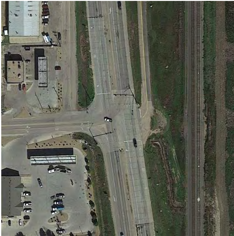
Figure 121 Aerial Photo: US 85C / SH 66 (MP 250.65)
