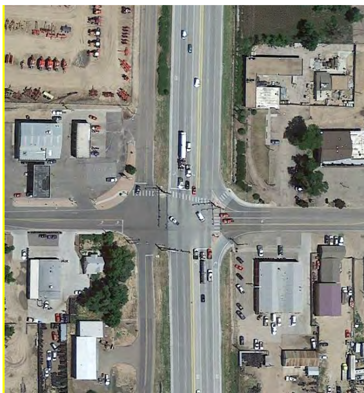
Figure 159 Aerial Photo: US 85L / US 34D (18 th Street) (MP 267.18)
