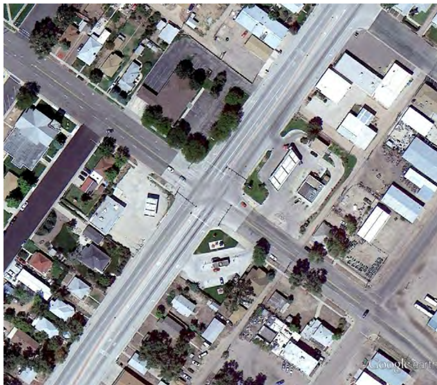
Figure 135 Aerial Photo: US 85C / SH 375 (1 st Avenue) (MP 262.63)
