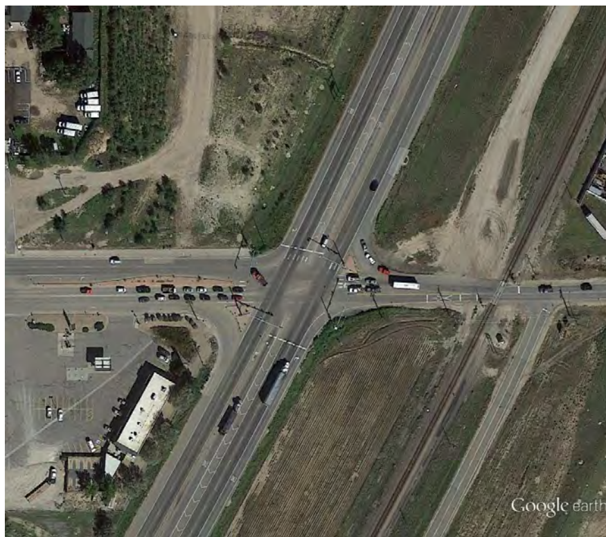
Figure 65 Aerial Photo: US 85C / 120 th Avenue (MP 229.76)
