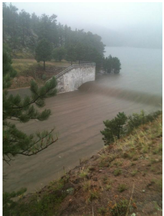
Spillway overflow at the Button Rock Dam
