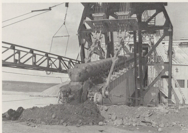
Figure 18. Bow of the South Platte No. 1 dredge, Each buckets' capacity was 13 cubic feet. (Colorado Historical Society, Zellars Collection)
