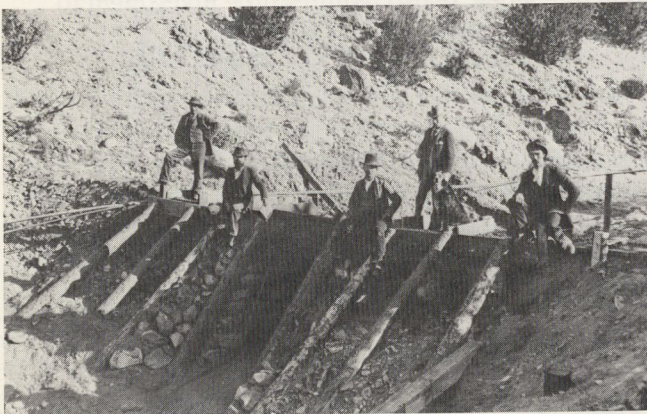
Figure 10. These men are posed on a dam built for booming. Note the gate in the middle that permits very rapid discharge of the dam. (Colorado Historical Society)
