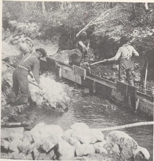
Figure 6. Miners feeding gravel into sluice. Note the "shoveling boards," used so that the miners can easily throw gravel into the sluice boxes with their shovels. (Colorado Historical Society)
