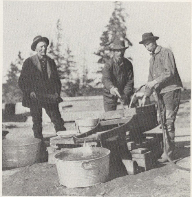
Figure 4. Men cleaning placer concentrates with rocker. (Colorado Historical Society)
