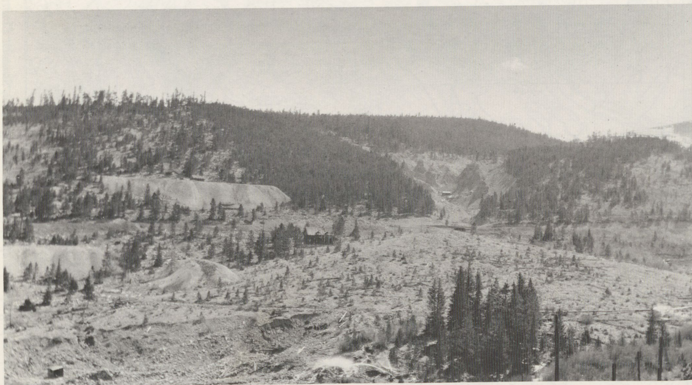
Figure 39. An historical photo looking northerly across Illinois Gulch toward Mayo Gulch, Breckenridge district, Summit County. The floor and lower walls of Mayo Gulch were placered—probably both boomed and hydraulicked. A fan of tailings was deposited in Illinois Gulch in which a monitor is cutting gravels in the foreground. (U.S.G.S. Photo Library, T. S. Lovering, 240)
