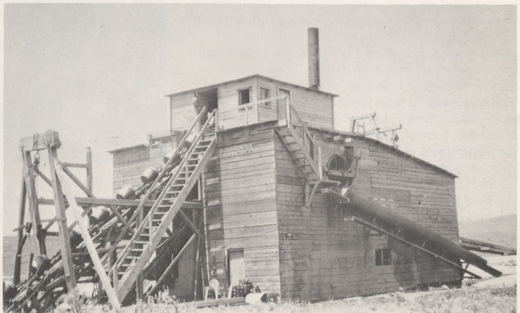
Figure 25. Blevins dredge, Iron Springs Divide, Moffat County. Many of the early dredges apparently were designed locally and much of their machinery made locally. Note the small buckets in the bucket line. The placer gravel in the Iron Springs Divide district contained few fragments larger than pebbles, and this dredge worked satisfactorily several seasons. (U.S.G.S. Photo Library, Gale, H. S. 303)
