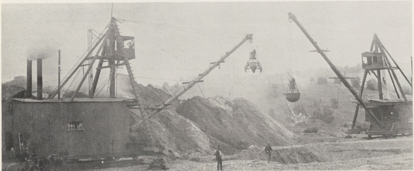
Figure 23. Two clam shell excavators built on site and used on the lower Blue River, Breckenridge district, Summit County, about 1900. These machines had capacities too small and slow to economically work the moderate grade gravels and could not move large boulders nor clean bedrock well. Note the wooden structures and the stacks indicating steam power. This was one of the methods attempted to work deep stream gravels before dredges were introduced. (Denver Public Library, Western History Department)
