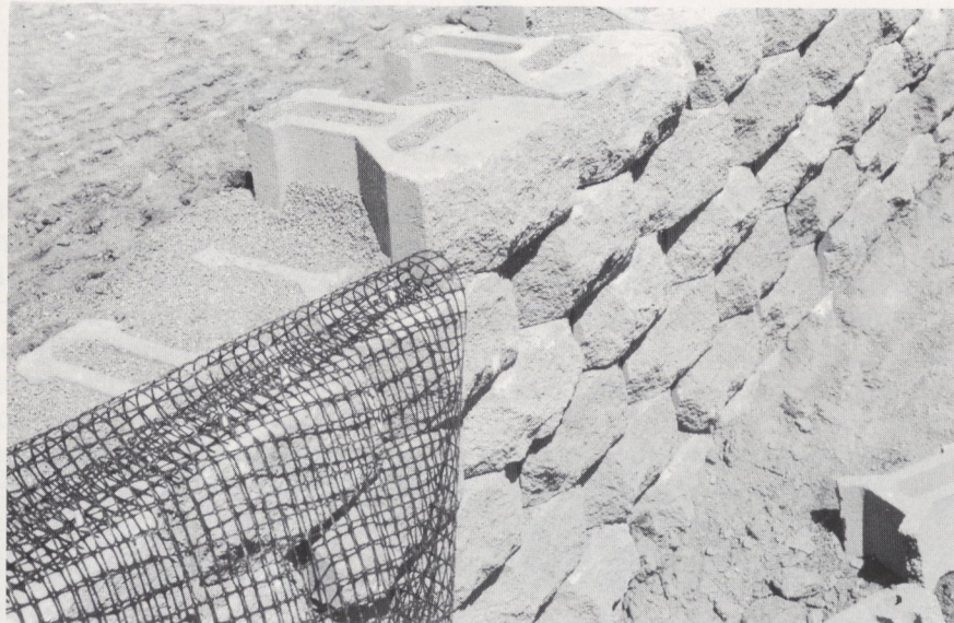
A completed Keystone wall.
